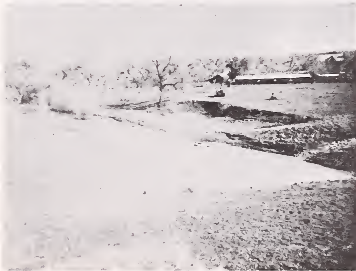
Photo No. 5.—1/27/69 10:32 a.m. Spillway stopped flowing.
